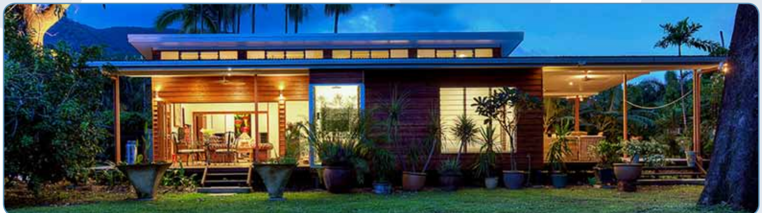
Verandas and good overhangs keep the home cool Chris Vandyke Designs. Photo: Sean Reason
