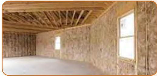
Wall insulation batts 2
