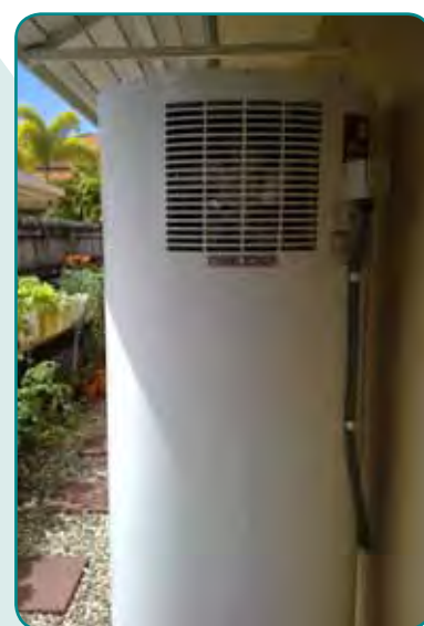
Heat Pump Hot Water System NQ Solar
